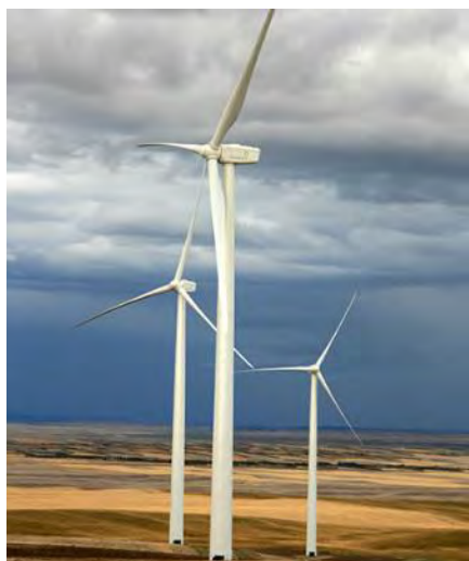
Utility-scale wind turbines. Photo Credit: WINDEXchange, U.S. Department of Energy
