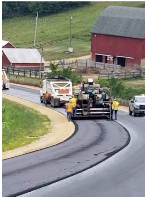
Rural road paving. Photo Credit: Jackson County Engineer
