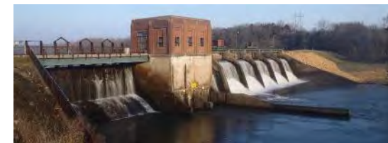
Maquoketa hydroelectric power plant. Photo Credit: http://renewableworldenergies.com
